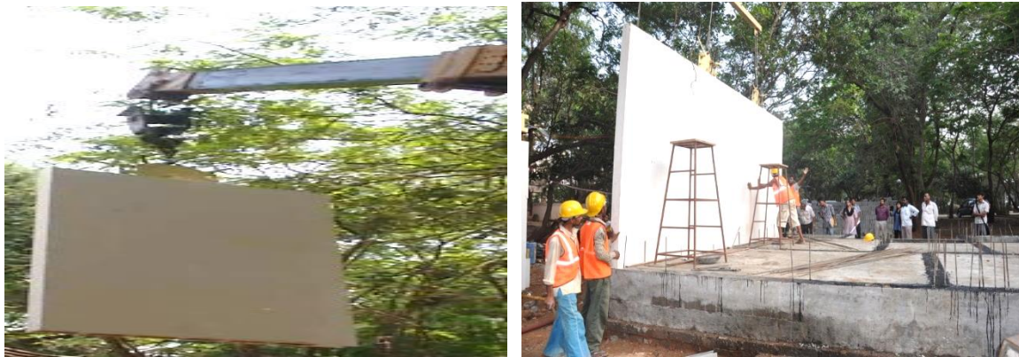
Figure 36: Lifting and placing of panels
