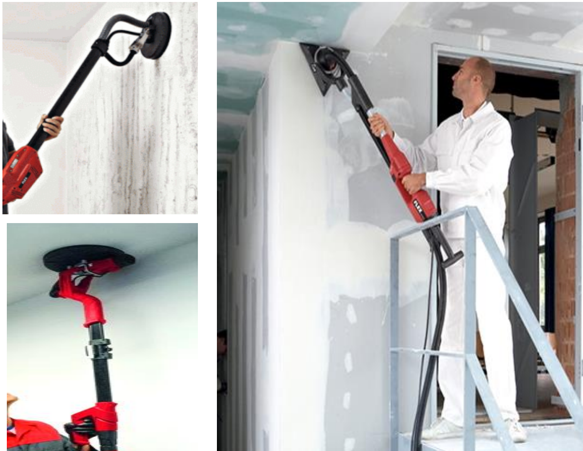
Figure 79: Grinding of wall panel surface using giraffe grinder
