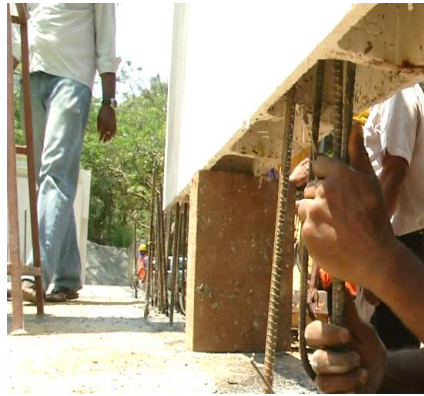
Figure 25: Wooden block for supporting wall panel
