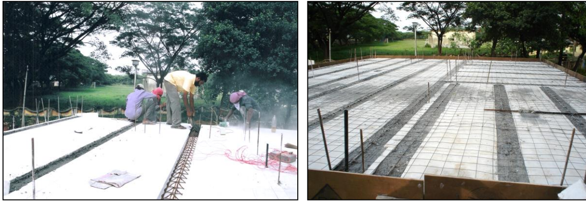
Figure 71: Concreting of concealed beams
