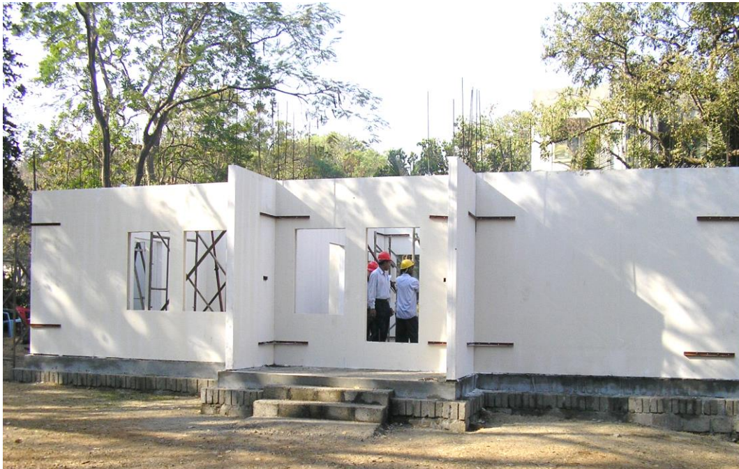
Figure 30: Wall corners held firmly using C-clamps / L-angles
