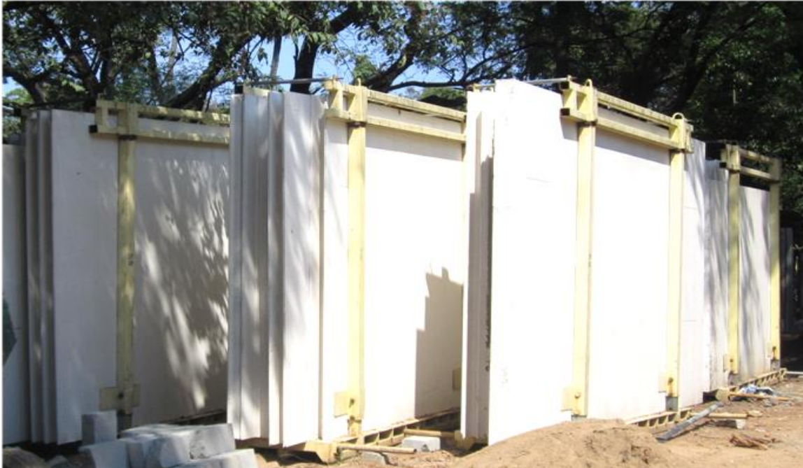
Figure 11: Panels stacked in stillages at construction site
