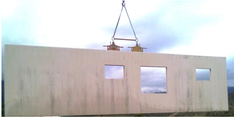
Figure 35: Lifting of long panels using lifting jaws and spreader bar
