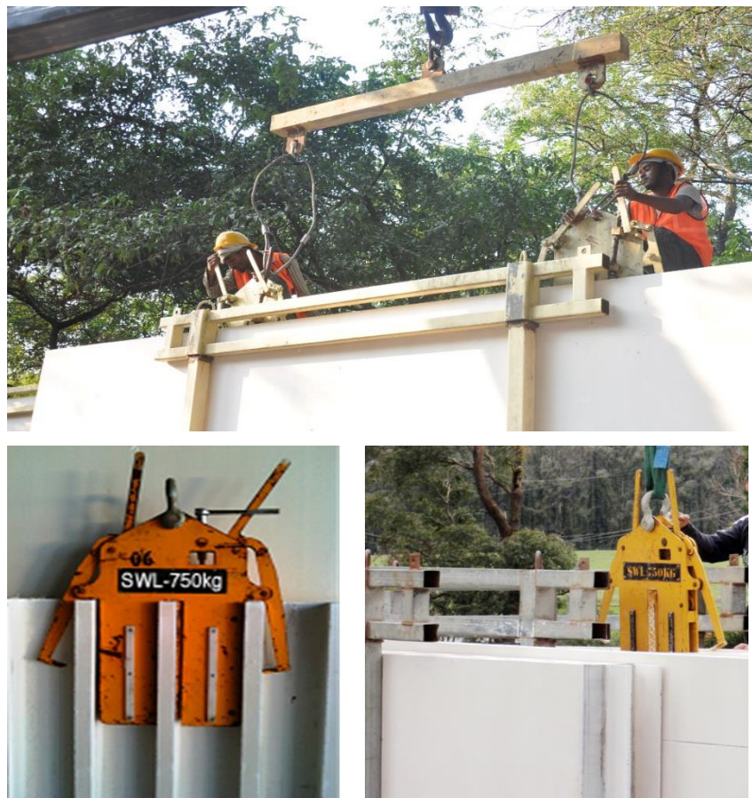
Figure 34: Identifying the panel based on notation mark and fixing the lifting jaws
