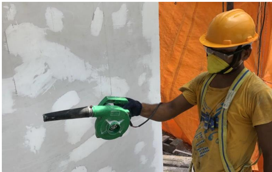
Figure A13.3 Blower used along with grinder to blow away the fine gypsum dust
