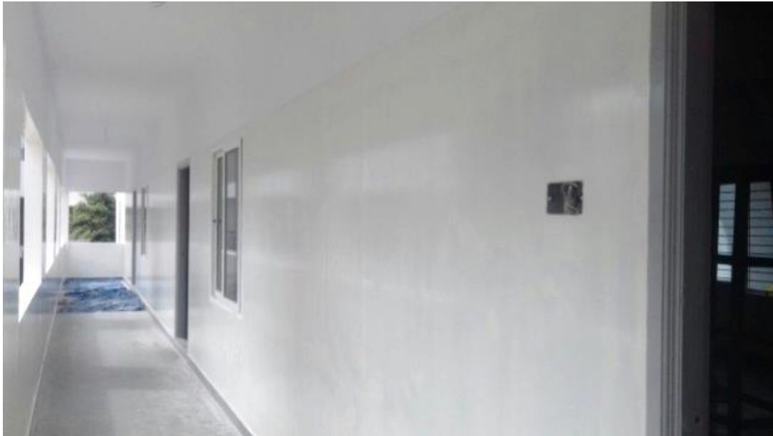
Figure A13.5 Finished wall surface of GFRG school building at Guindy, Chennai, after application of finishing coat of paint (before rendering)
