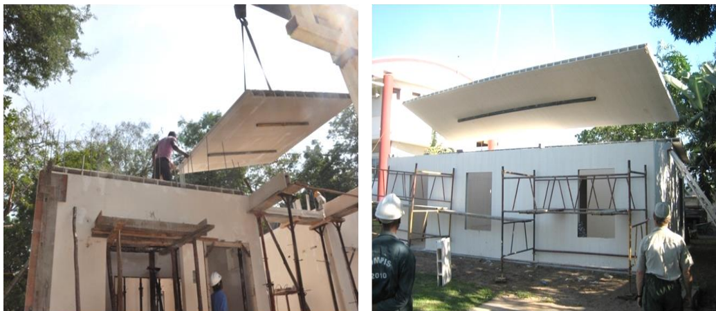
Figure 64: Lifting of slab panel in horizontal position using under panel spreader bar and sling rope
