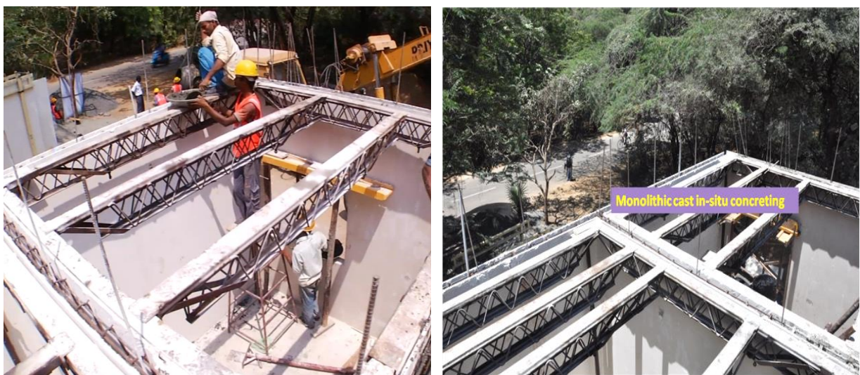
Figure 63: Support system for laying floor slab panel in position
