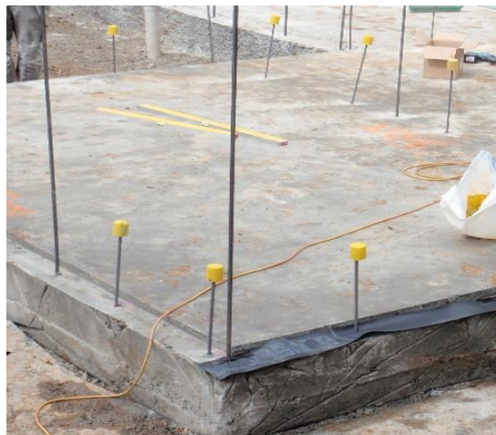
Figure 19: Completed foundation with starter bars in position (a) wrong practice (b) right practice
