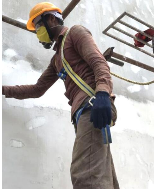
Figure A13.2 Patching of dents on walls and 174 / 184 mm wide band using water resistant patching compound / rendering compound, by a putty applicator
