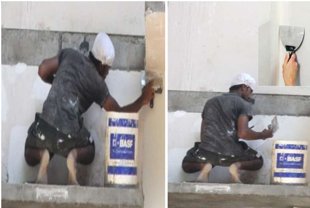
Figure 82: Rendering of GFRG wall panel surface using Rapidwall plaster mix
