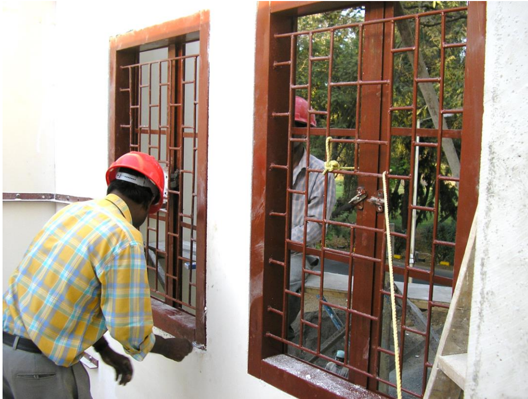
Figure 51: Installation of window frames
