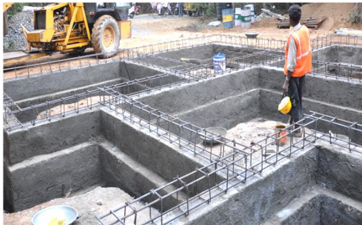
Figure 17: Reinforcement for RC plinth beam
