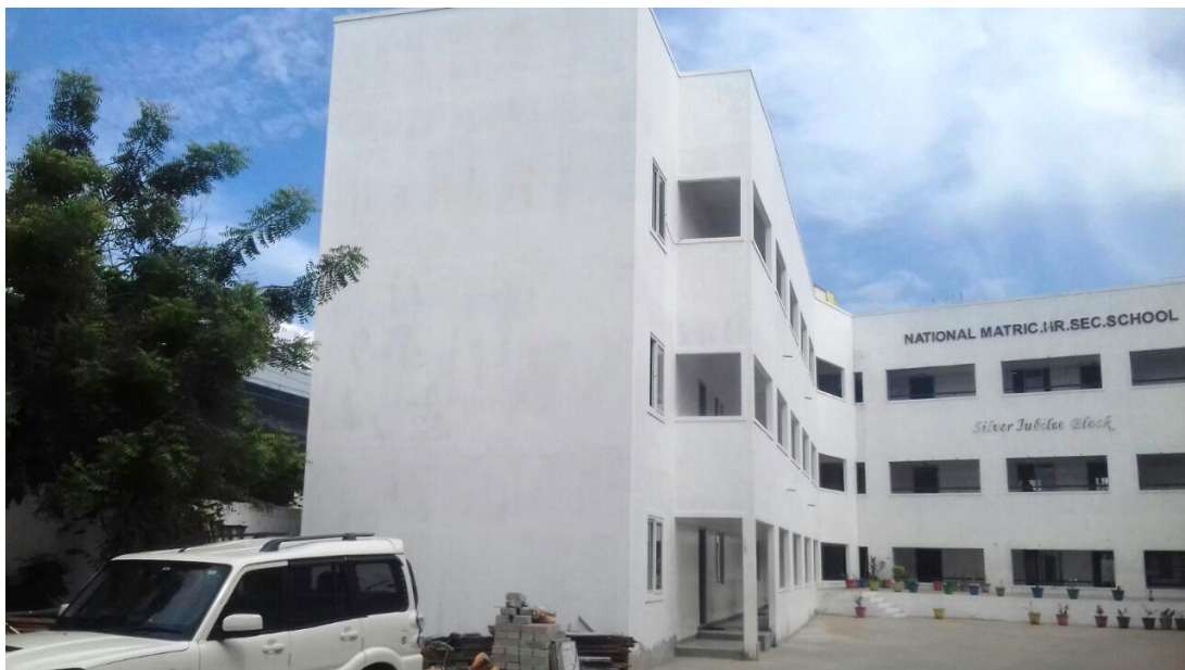
Figure A13.6 Front view of the GFRG school building; after application of special primer, finishing of patching work, grinding of 174 / 184 mm wide band using wood grinder and filling-up to level and smoothen the surface and painting, without rendering
