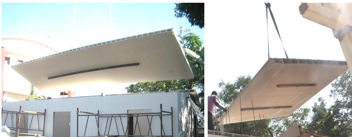
Figure 24: Under panel spreader bars
