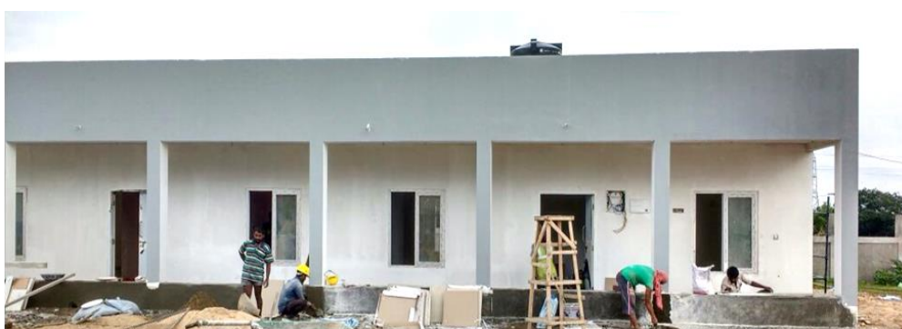
Figure A13.8 Rendering (using water-resistant rendering compound) being carried-out for the maintenance building of IIT Tirupati
