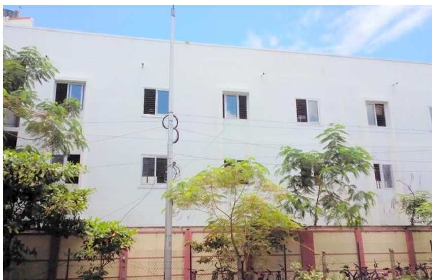
Figure A13.7 Rear view of the GFRG school building at Guindy, Chennai, before rendering
