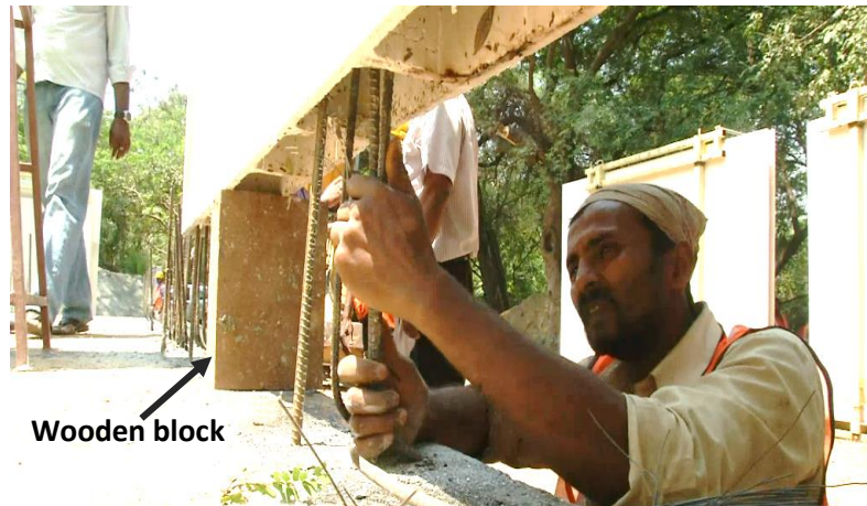
Figure 37: Tying of starter bars with the vertical bars while erecting panel
