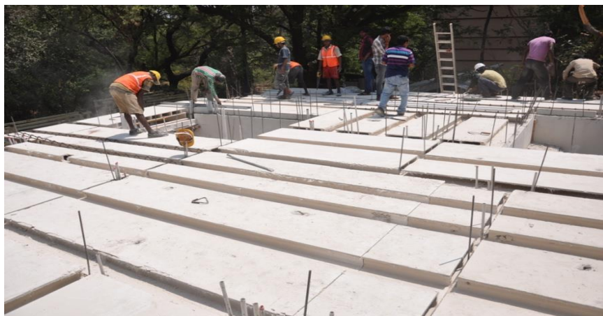
Figure 66: Flanges cut open for casting concealed beams
