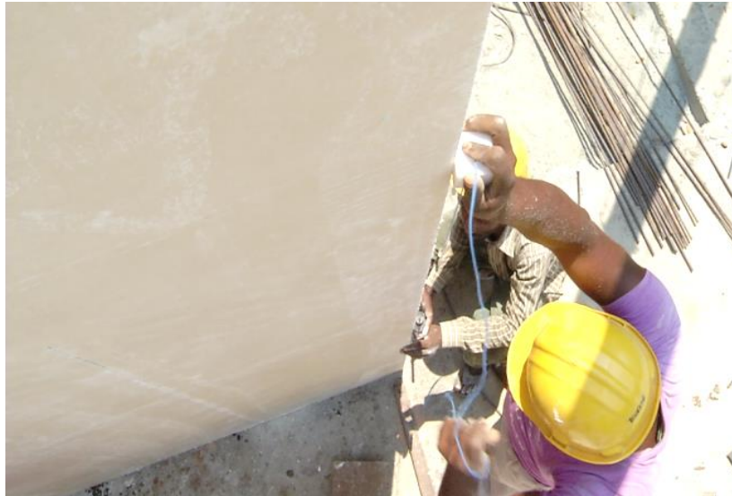
Figure 39: checking of vertical plumb
