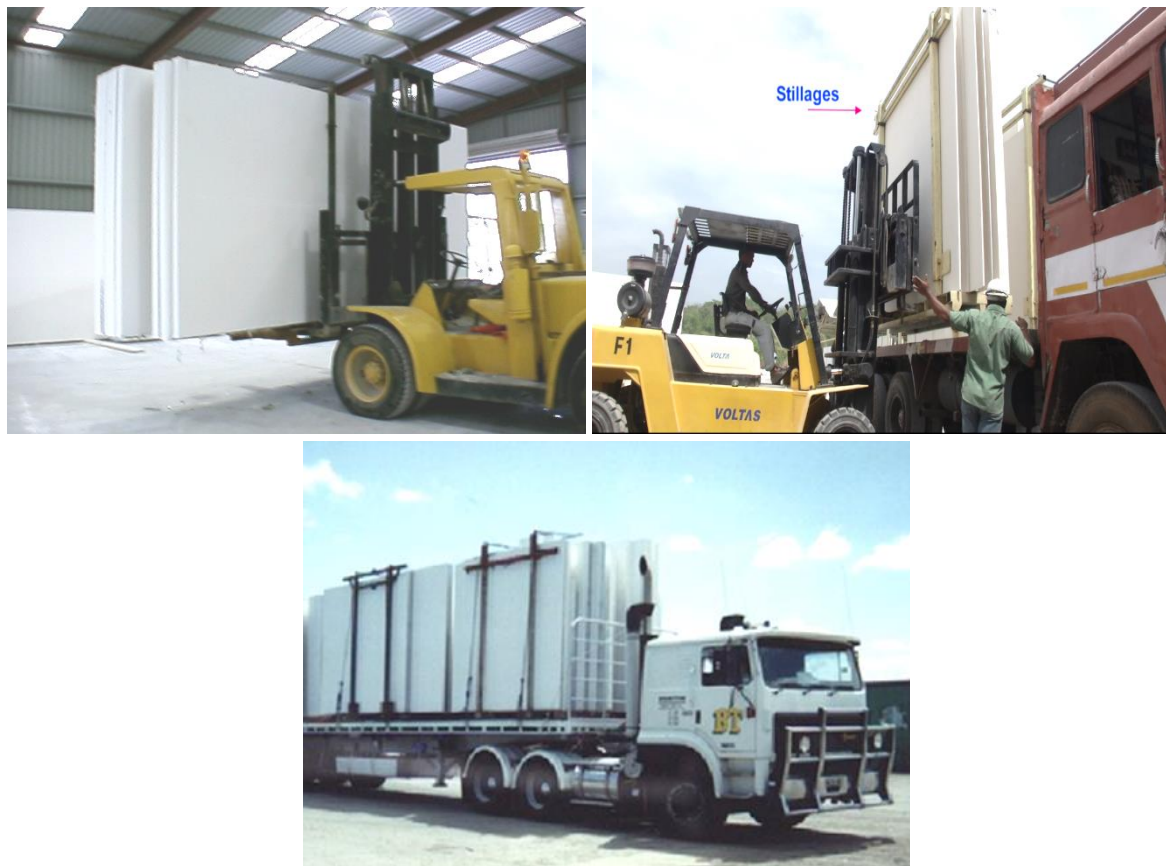
Figure 10: Loading and transportation of GFRG panels
