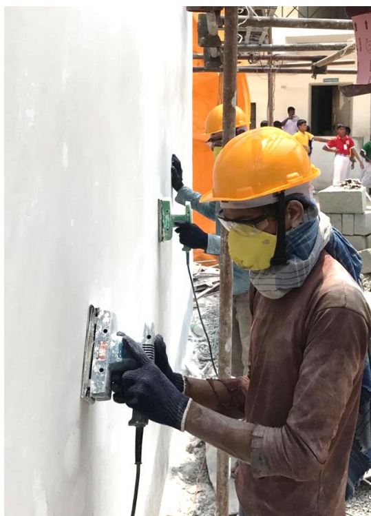
Figure A13.4 Putty applicators grinding the patched-up spots / areas for levelling and smoothening, using wooden grinder with sandy disc
