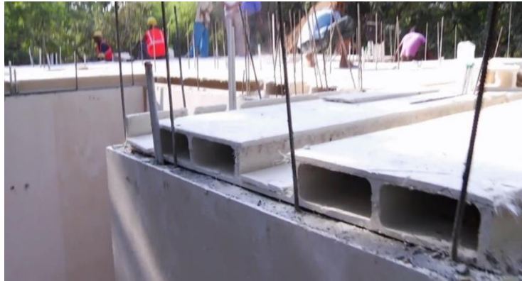
Figure 65: Bearing of slabs over walls
