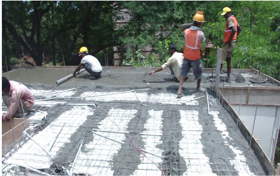
Figure 72: Concreting of slab
