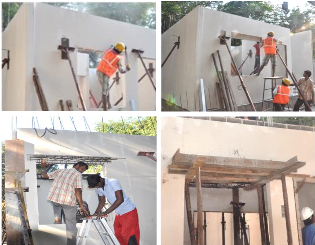
Figure 49: Providing RC lintel cum sunshade
