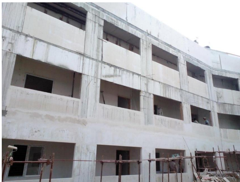
Figure A13.1 Three storeyed GFRG school building at Guindy, Chennai (constructed in 2017), after the required waterproofing treatment and application of mandatory primer
