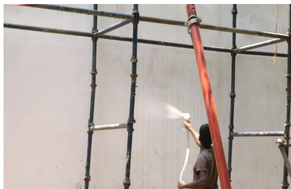
Figure 78: Spraying of primer on GFRG panel surface
