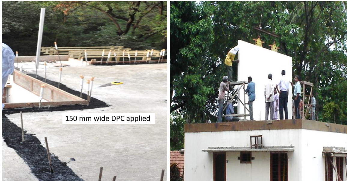
Figure 75: Application of DPC and erection of wall panel
