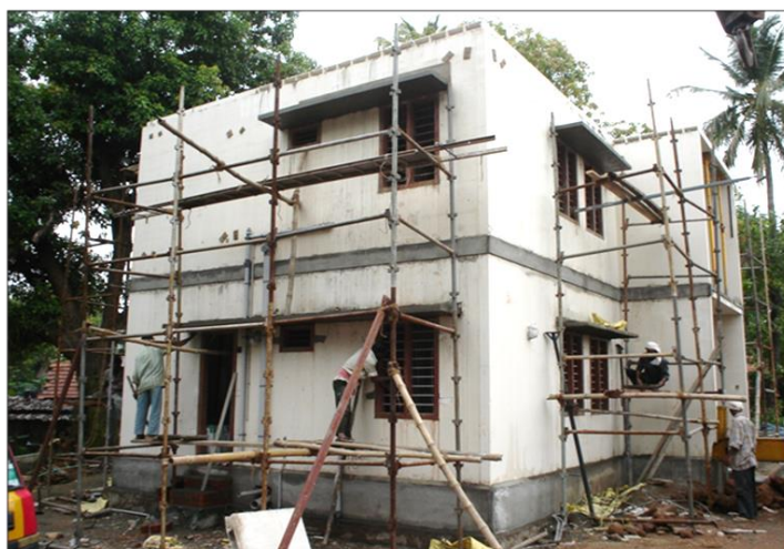
Figure 76: Scaffolding provided for a GFRG building
