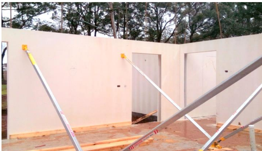
Figure 40: Lateral props fixed tightly and the panel in rigid position
