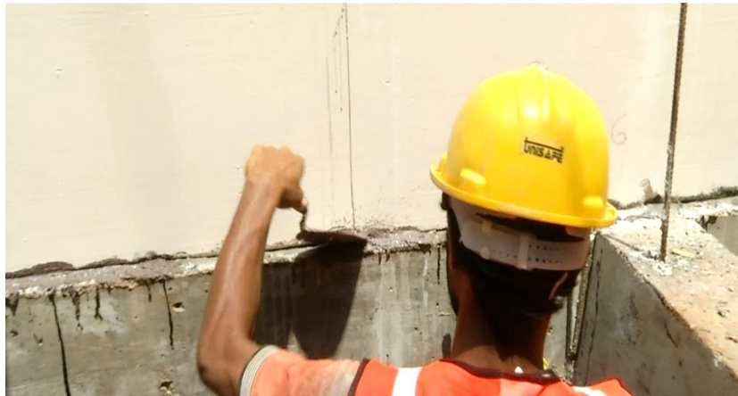
Figure 41: Sealing-off of joint with joint sealant
