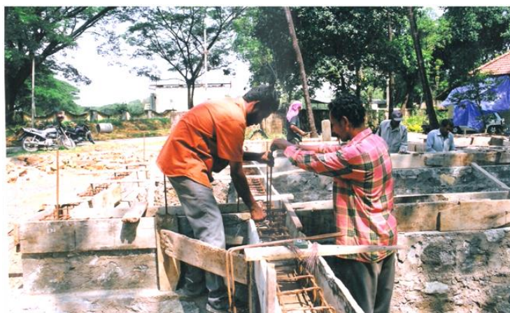
Figure 18: Inserting starter bars
