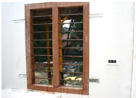
Figure 77: Windows and switch boxes fixed on to panel
