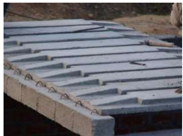
Figure 15: PRE-CAST RCC PLANK AND JOIST
