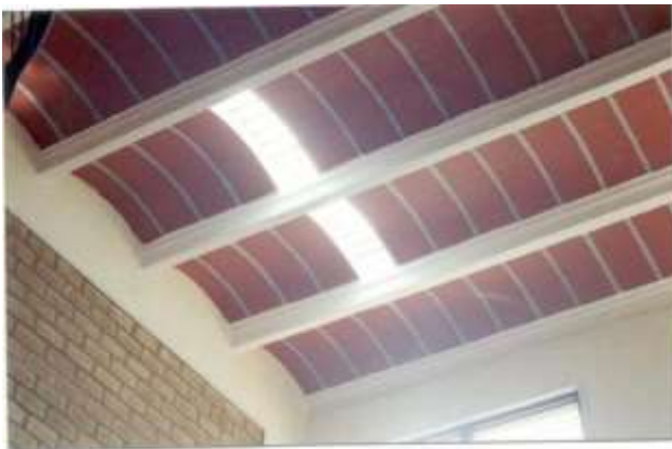
Figure 16: PRE-CAST ARCH PANEL SYSTEM
