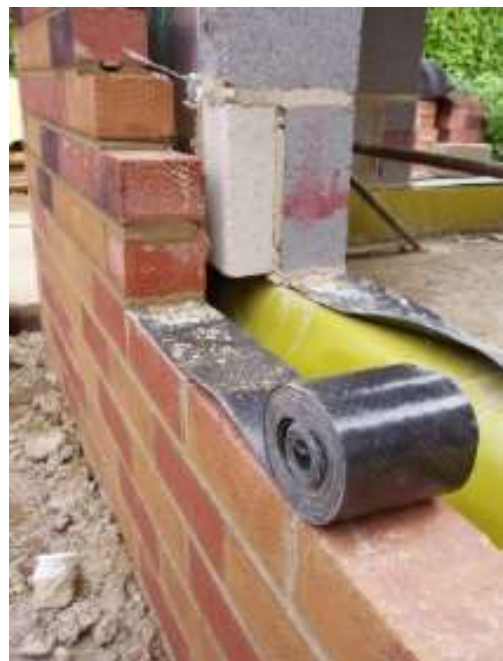
Figure 20: DAMP PROOF MEMBRANE
