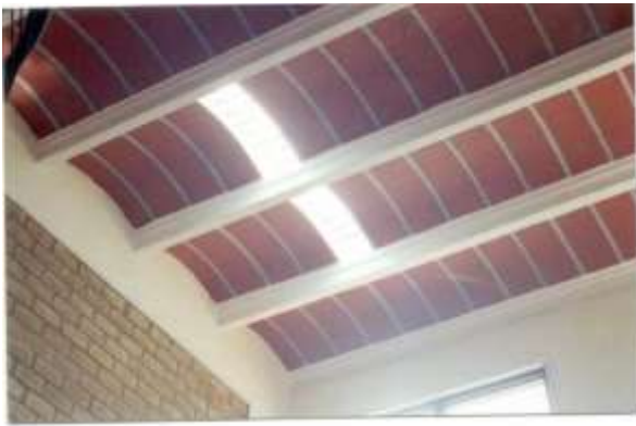
Figure 16: PRE-CAST ARCH PANEL SYSTEM
