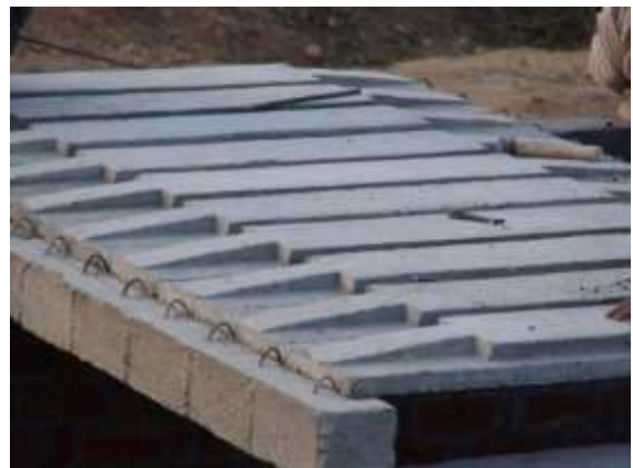
Figure 15: PRE-CAST RCC PLANK AND JOIST
