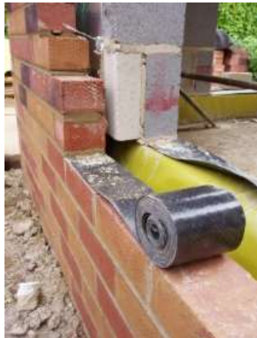
Figure 20: DAMP PROOF MEMBRANE
