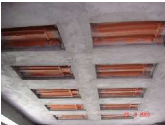
Figure 14: FILLER SLAB
