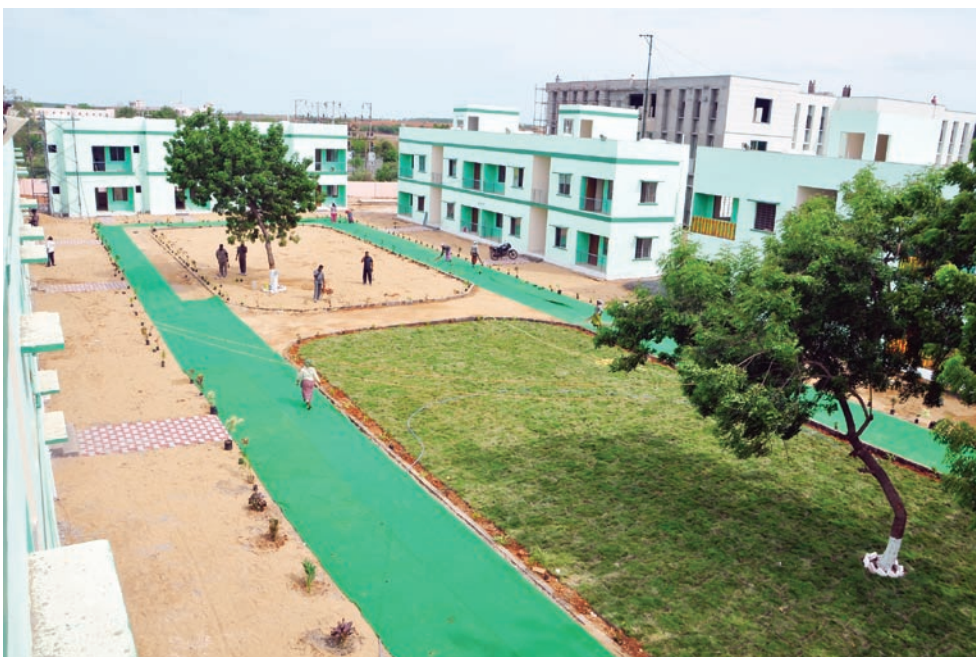
Demonstration Houses (36 DUs) constructed using Glass Fibre Reinforced Gypsum (GFRG) Panel System at Nellore, Andhra Pradesh
