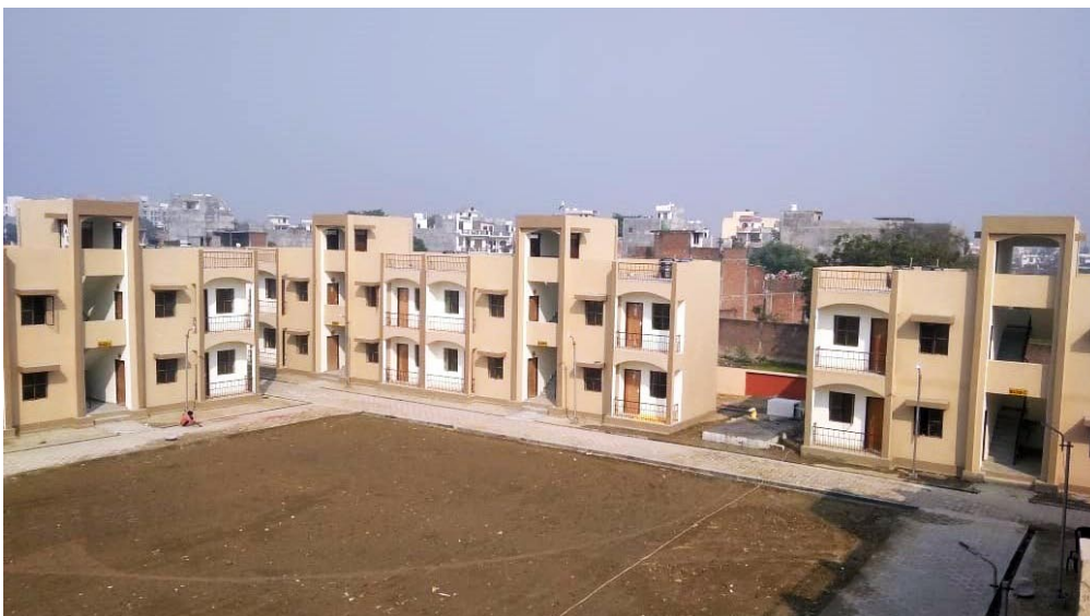
Demonstration Houses (40 DUs) constructed using Stay in Place Double Walled EPS Panel System at Aurangabad Jagir, Lucknow, Uttar Pradesh
