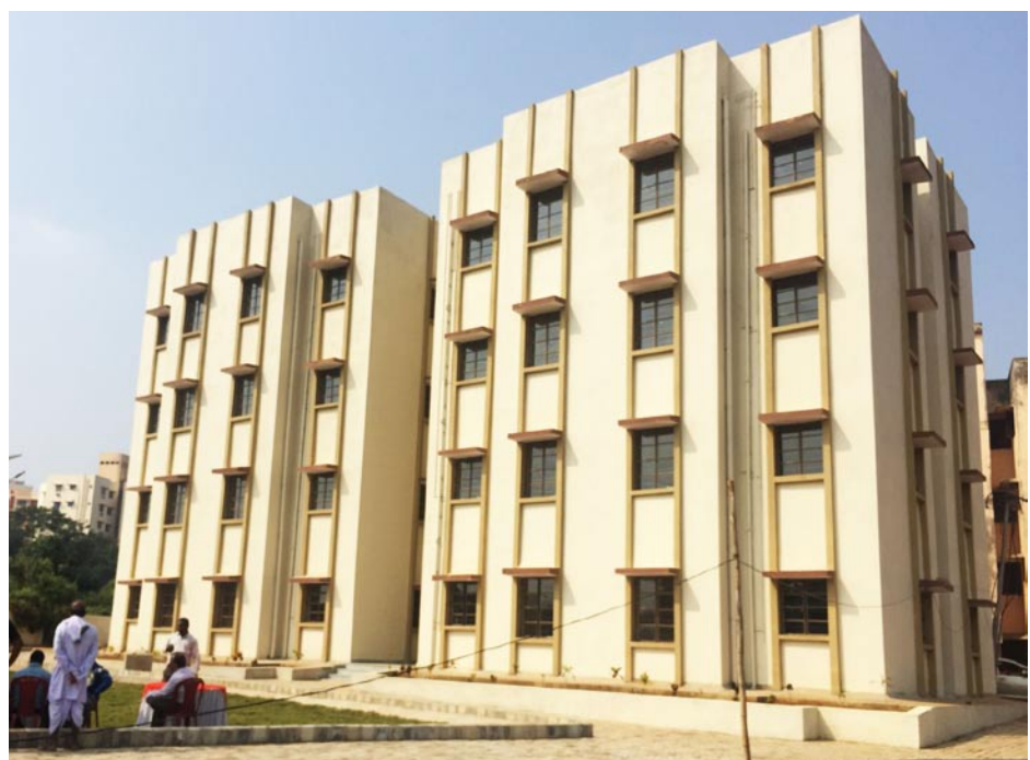
Demonstration Houses (32 DUs) constructed using EPS Core Panel System at Bhubaneswar, Odisha
