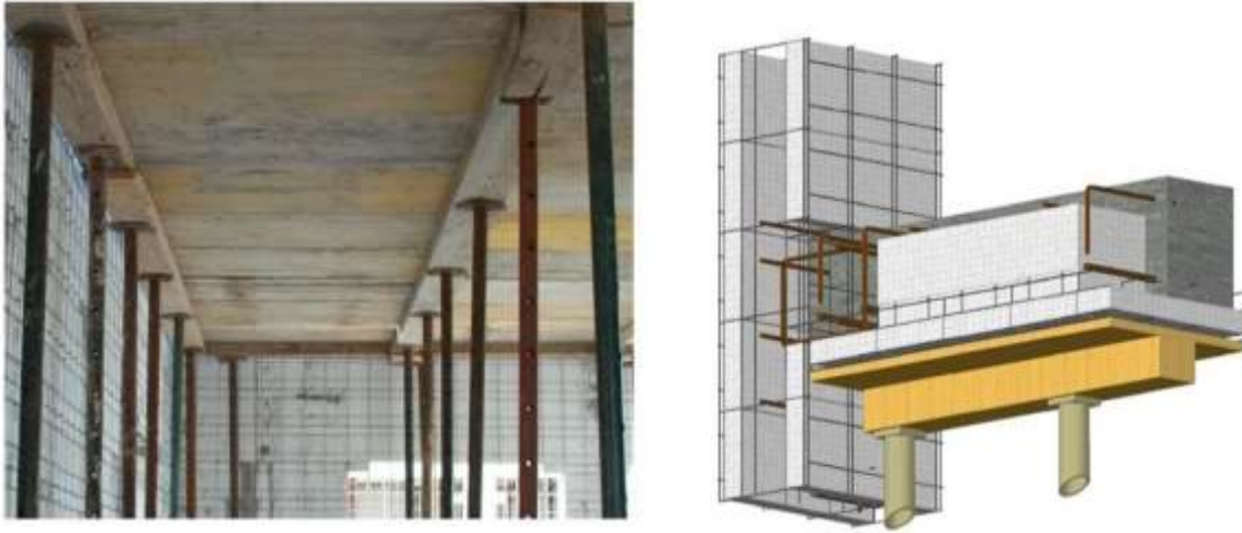
Fig. 22 & Fig. 23 Floor props supporting beams and shuttering board Placing of reinforcement
