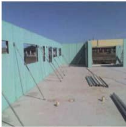
Fig. 8 Diagonal bracing
