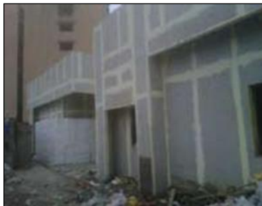
Fig.12 Yellow Putty with Fibre mesh tape
