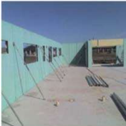
Fig. 8 Diagonal bracing
