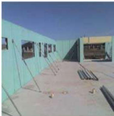
Fig. 4 Diagonal bracing
