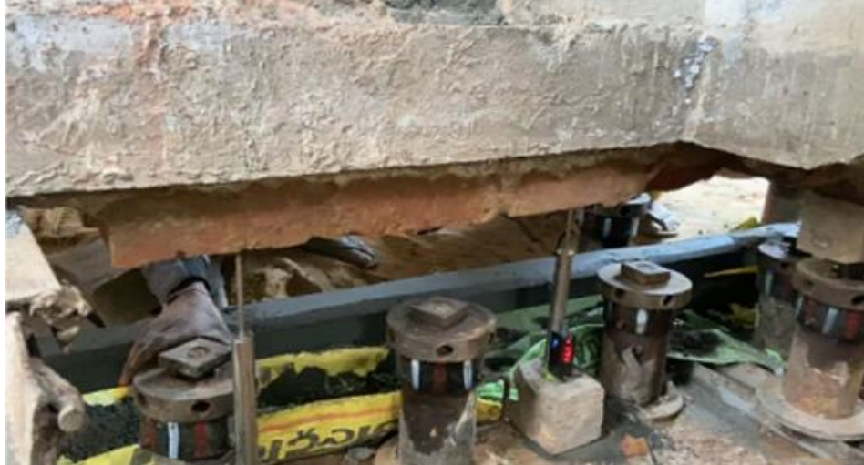
Fig. 6: LVDT placements below the selected region of the wall
