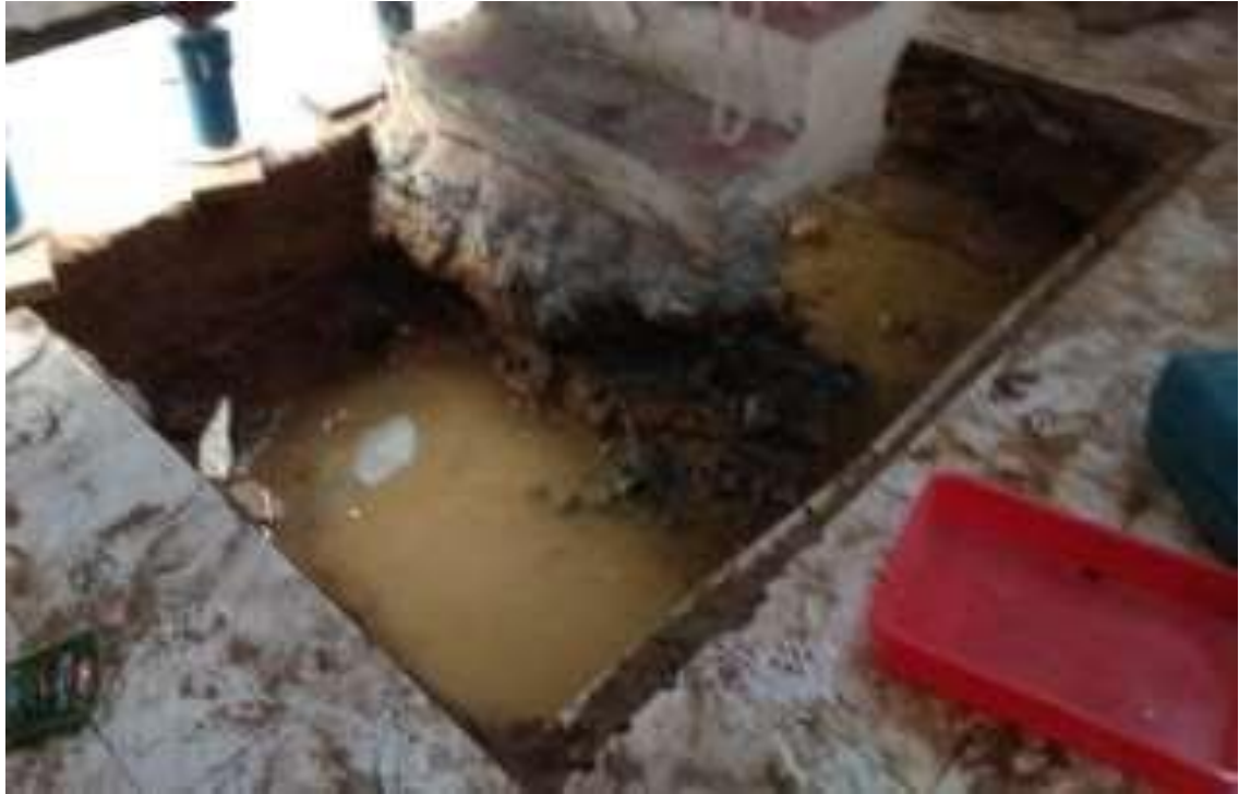
Fig. 1: Excavation of foundation
