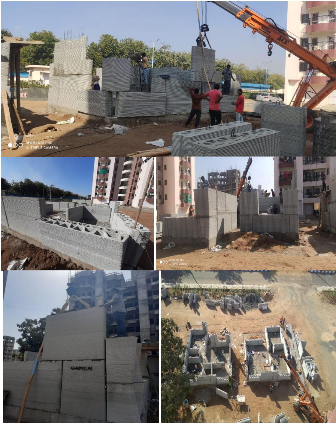
Fig. M10 Assembly of modules
