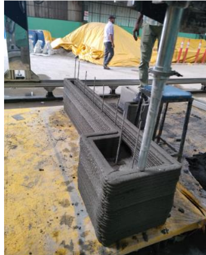
Fig. M8 Printing around the bars
