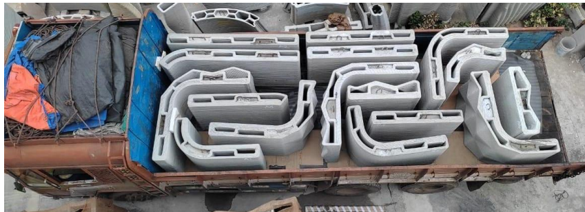
Fig. M9 Transportation of modules
