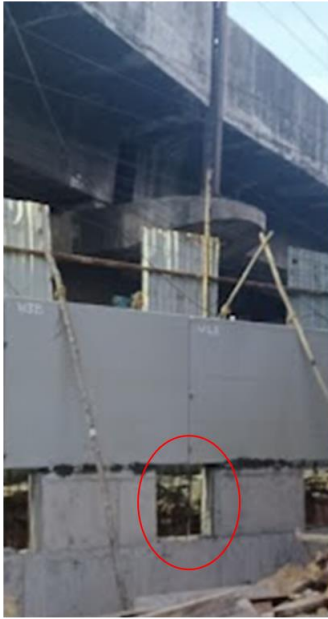
Provision to Join panels with footing wall/ plinth beam
