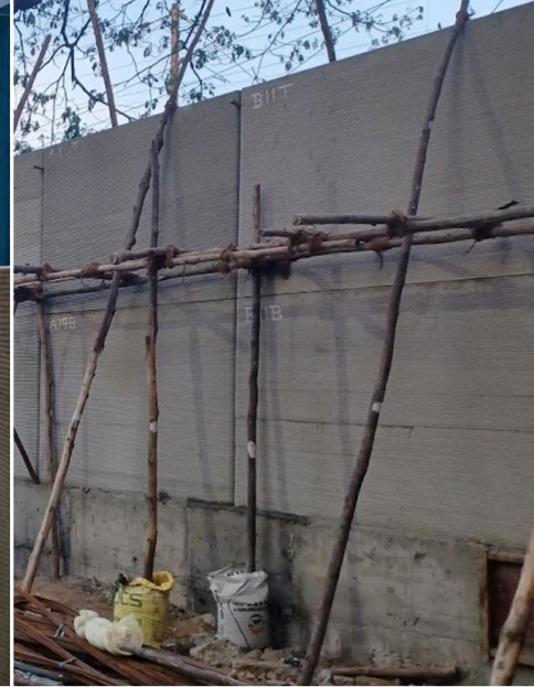
Lateral support during grouting of column/beam
