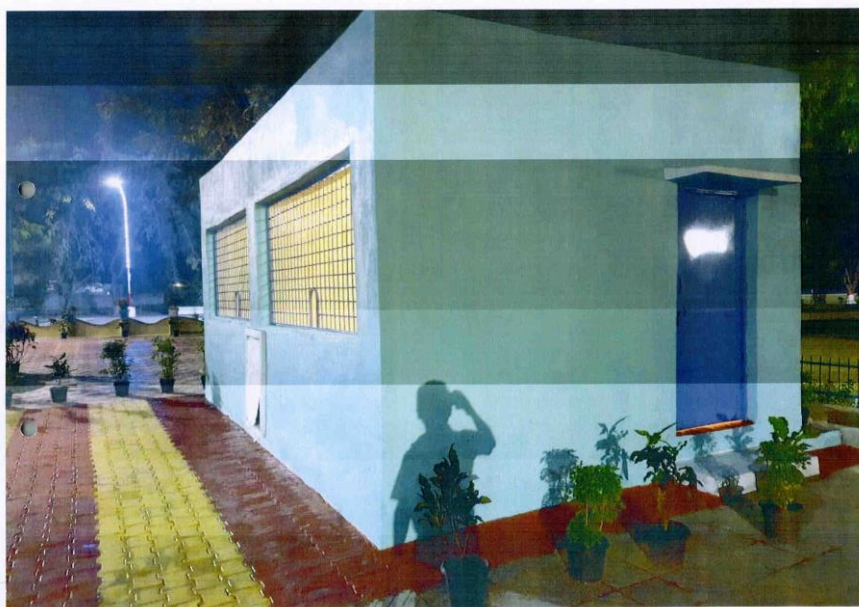
Model building constructed using GPCA at NTPC Ramagundam
