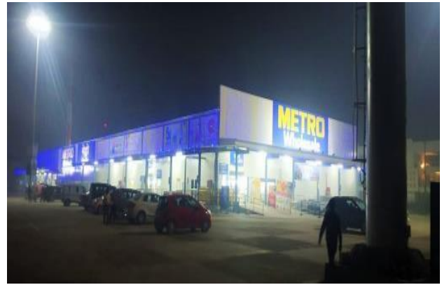
Warehouse Building (PEB), Aditya Moda, Ghaziabad
