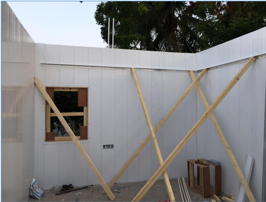
Panel bracings with aluminum angle
