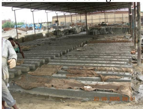
Fig.31 Precasted joists under covered shed
