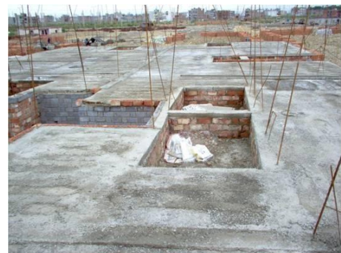
Fig.36 The sunk slabs and vertical reinforcement projecting out
