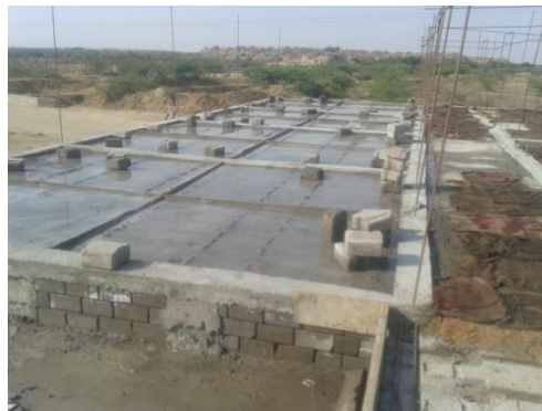
Fig.35 Filled up haunches with in-situ concrete (curing being done)
