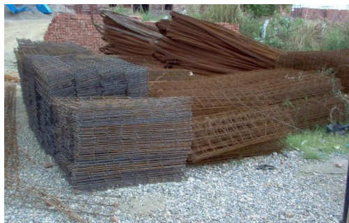
Fig.23 Stack of reinforcement cage for different size of planks
