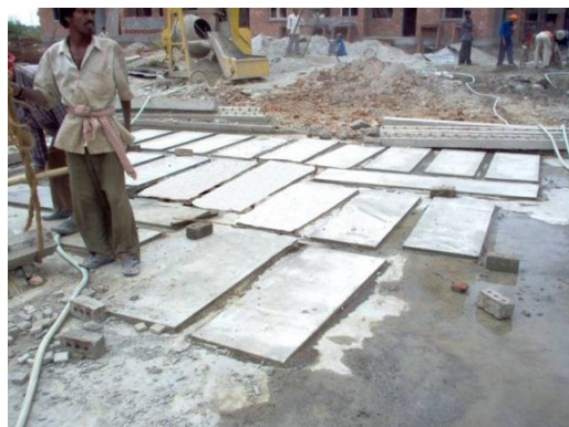
Fig.37 Precasting ferrocement shelves
