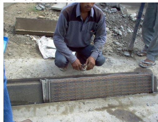
Fig.38 Mesh placed on mould (staircase steps)
