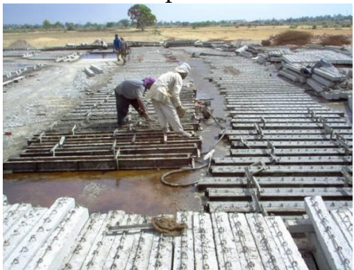
Fig.30 RC joists being precasted
