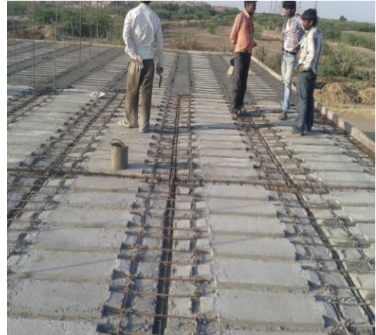
Fig.34 reinforcement in haunches
