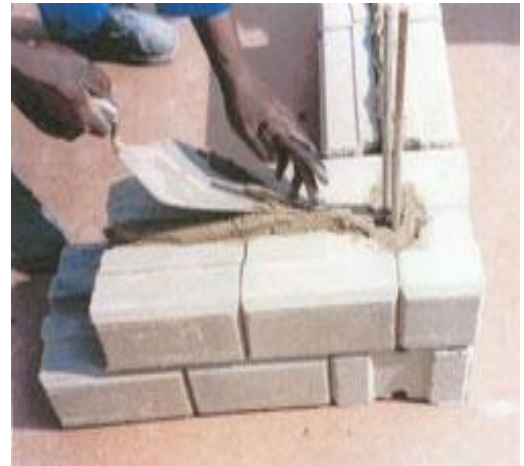
Fig.20 Corner vertical reinforcement
