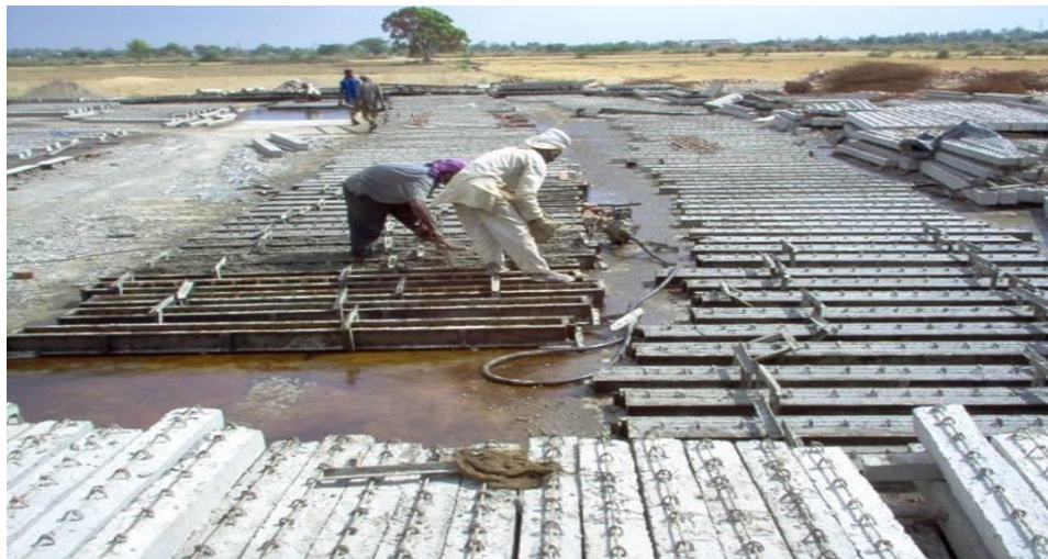
Fig. 12 – Precasting of joists with MS Channel molds
