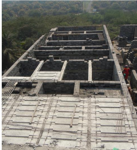
Fig.33 Planks & Joists being placed on walls
