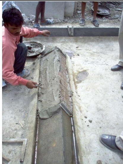
Fig.39 Laying mortar and finishing stairs step
