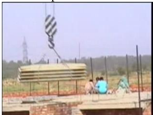
Fig.32 Lifting of planks mechanically
