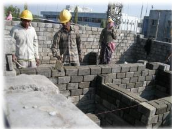
Fig.21 a,b,c,d walls under construction
