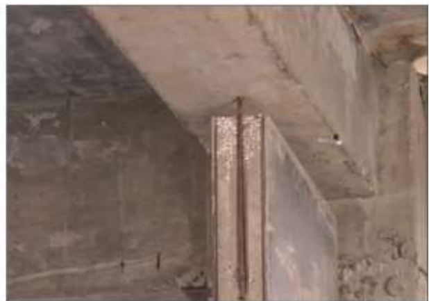
6. Planting Bars in Structure Beam
