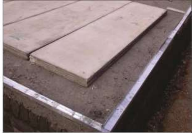
2. Fit the "C" Channel
