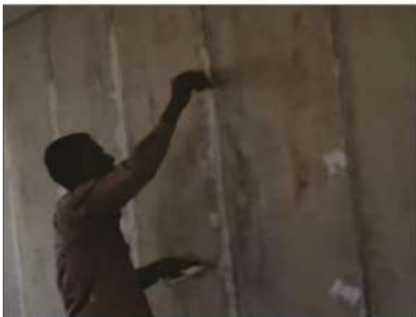
11. Grouting and filling starch
