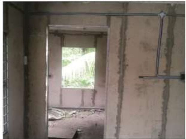
10 Installing electrical wires and switches
