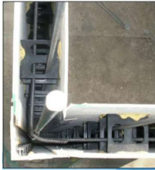
Top View of Plaswall at Corner Junction
