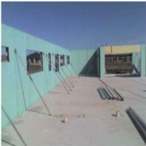
Fig. 13 Diagonal bracing
