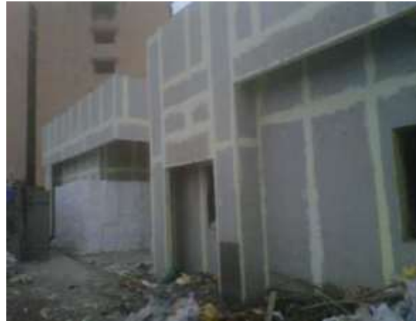
Fig. 17 Joint Treatment Fig. 18 Yellow Putty with Fibre mesh tape
