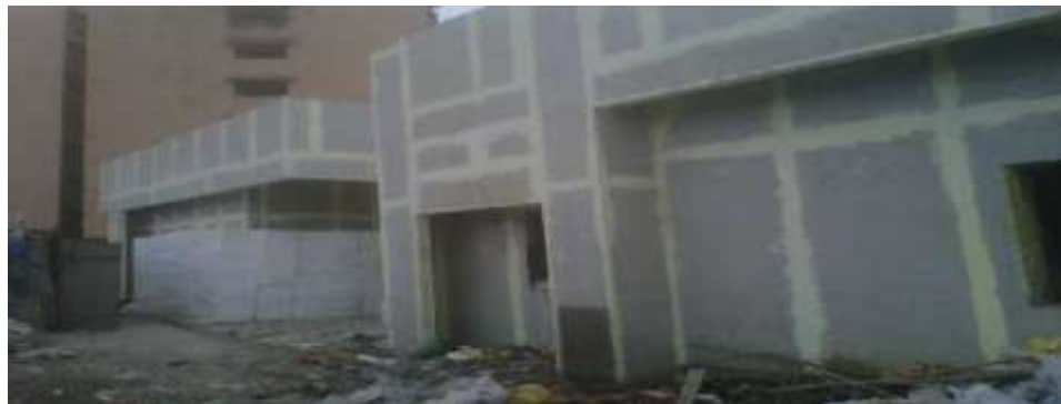
Fig. 30 Yellow Putty with Fibre Mesh Tape
