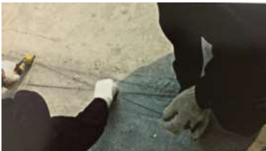
Fig. 3 Marking of the panels as per drawings
