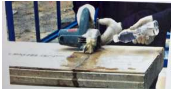
Fig. 4 Cutting of panels as per drawings
