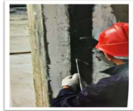
Fig. 6 Applying cement and glue
