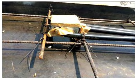
Fixing electrical boxes and conduits
