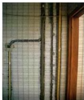
Fig. 71 Ducts embedded into concrete and/or insulation strips, either pouring concrete or afterwards in the insulation (cut or malt)
