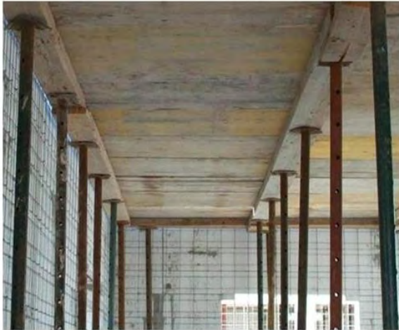
Fig. 36 & Fig. 37 Floor props supporting beams and shuttering boards
