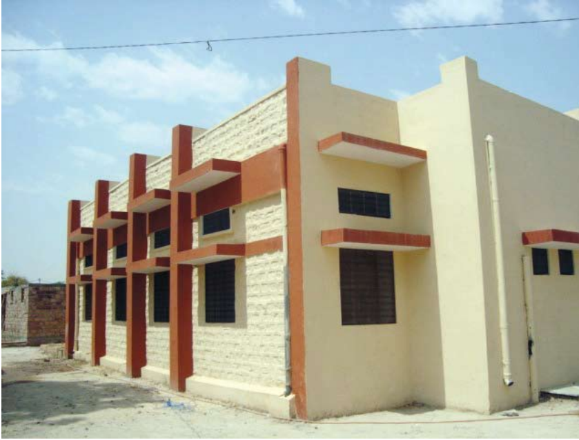
Community centre in insitu Up-Gradation site at Rajasthan
