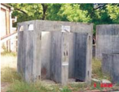
Service core unit (Bath & Toilet)
