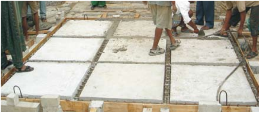
Construction of precast panel
