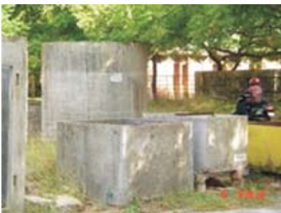
Circular(10000 liters) and rectangular Ferro-cement water tanks (1000 liters)
