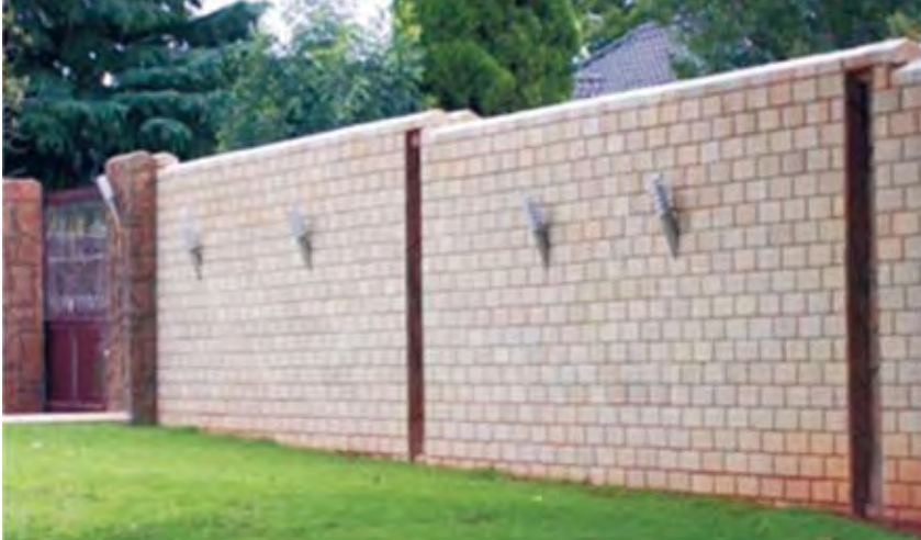
Figure 10: Boundary wall with Interlocking Blocks
