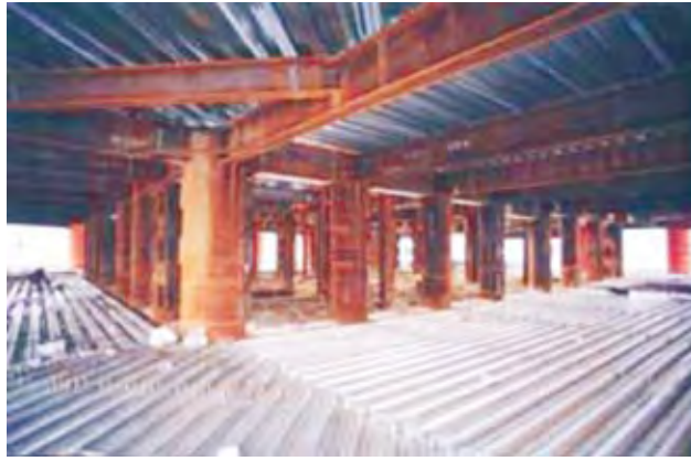
(a) CFT columns used in construction of SEG Plaza in Shenzhen, China, Height = 291.6 m
