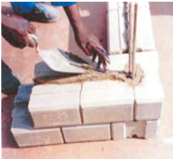
Figure 9: Vertical Steel in Masonry
