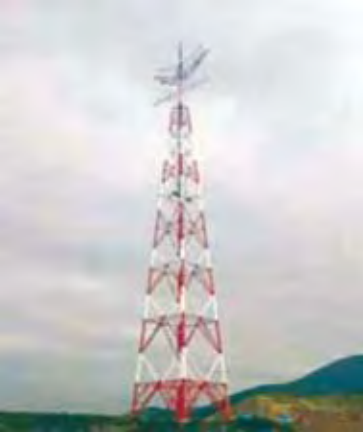
(b) A transmitting pole with CFT legs 370 m in height (China)
