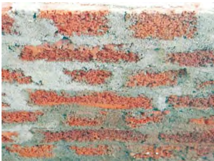
Fig.3 Partition wall made of LWFB
