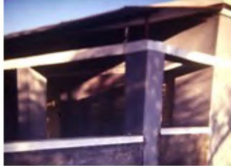
Seismic bands at lintel, roof and plinth levels
