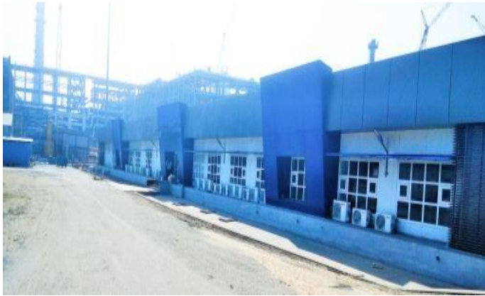
Field Maintenance Office, Reliance Industries Limited, Jamnagar
