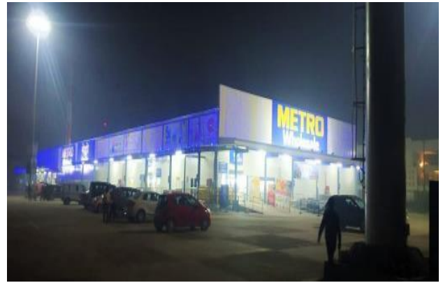
Warehouse Building (PEB), Aditya Moda, Ghaziabad
