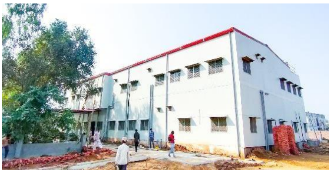
PEB G+1 Building, Dr Shroff Eye Hospital, Saharanpur, UP
