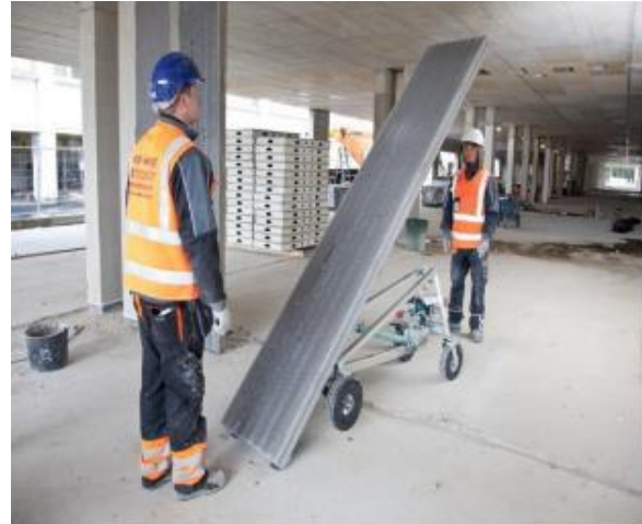
Unloading of panel
