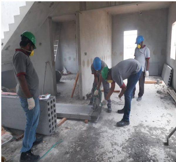
Drilling and cutting being done on Panels
