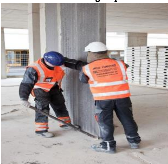
Tongue and Groove to be carefully positioned against each other
