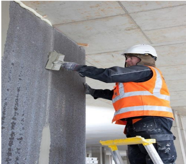
Gluing agent spreaded on side of the panel
