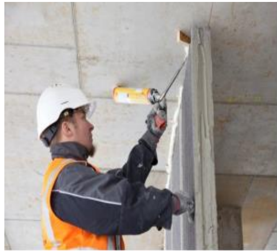
Top joint filled with PUF
