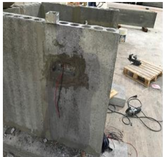
Fixing of Electrical fittings
