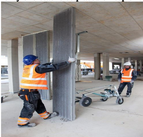
Panel are fixed to the floor & ceiling
