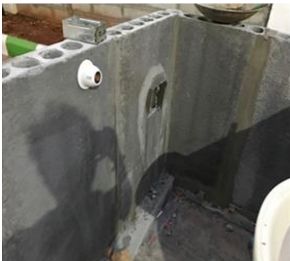
Fixing of Plumbing fittings
