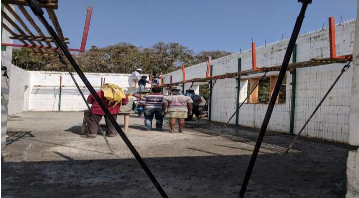
Scaffolding: Platform on trestles for access & assembly of high walls
