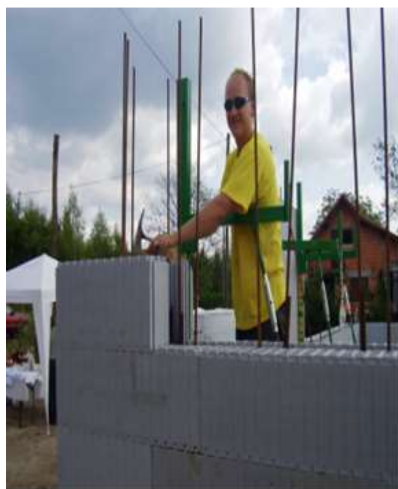
Installing Vertical re-bar
