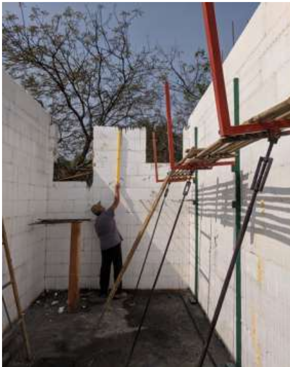
Bracing: support to the walls before concreting frames
