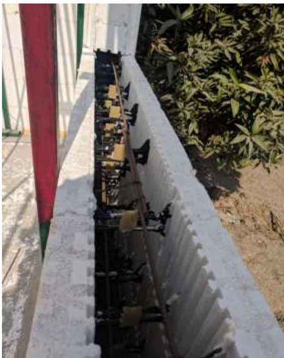
Inserting Horizontal Re-bars
