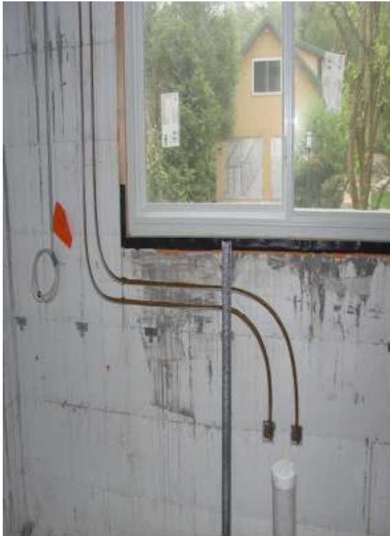
Conduits & Pipes: Inside chased lines
