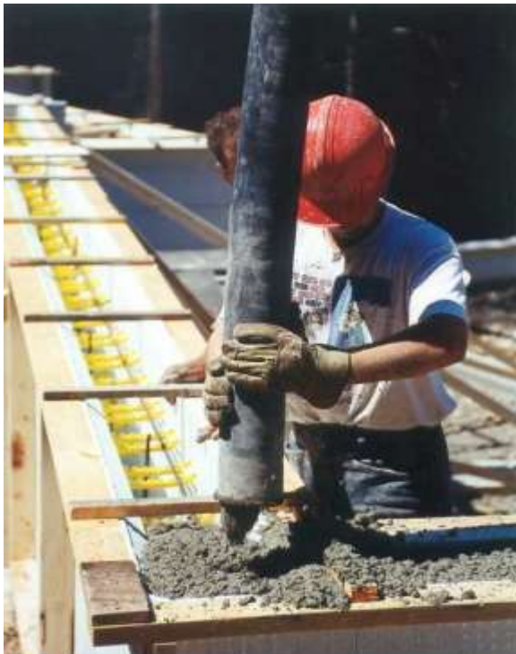
Concrete pouring: (High slump concrete poured inside formwork)
