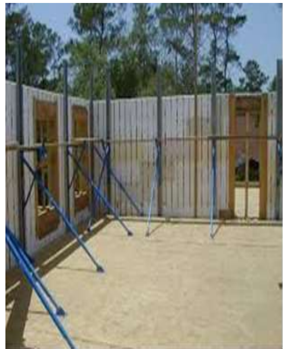
Propping: Fixing framework props around doors & window
