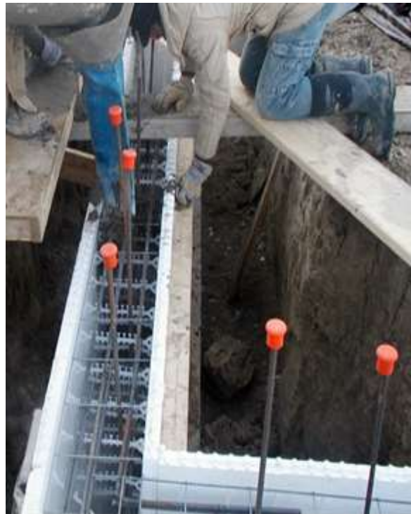
Concrete pouring: (High slump concrete poured inside formwork)
