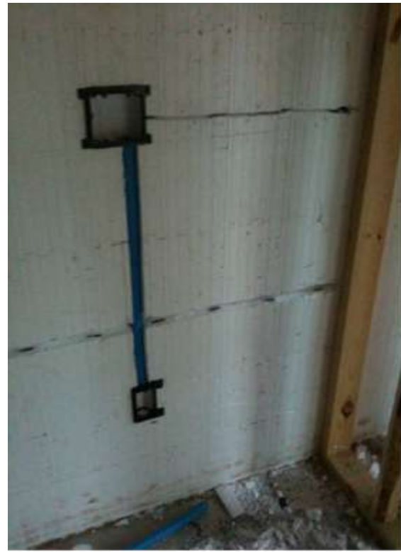
Conduits & Pipes: Inside chased lines
