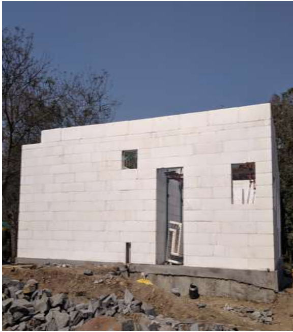
Insulated Walls: External walls
