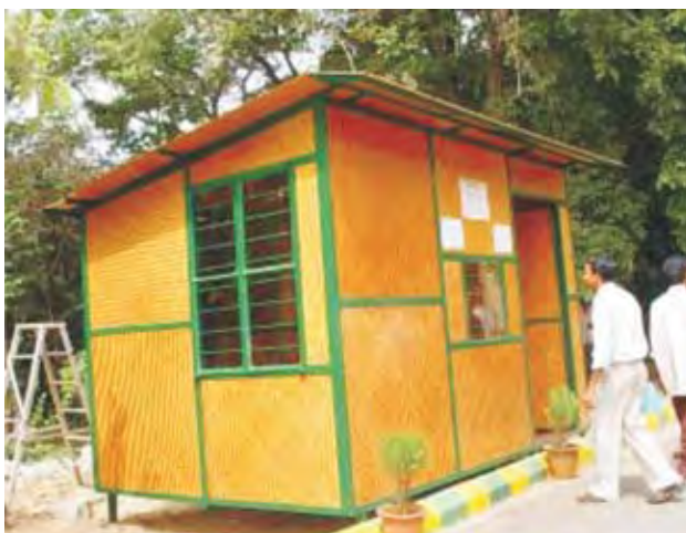
Plate 2 Steel Prefabricated Bamboo House
