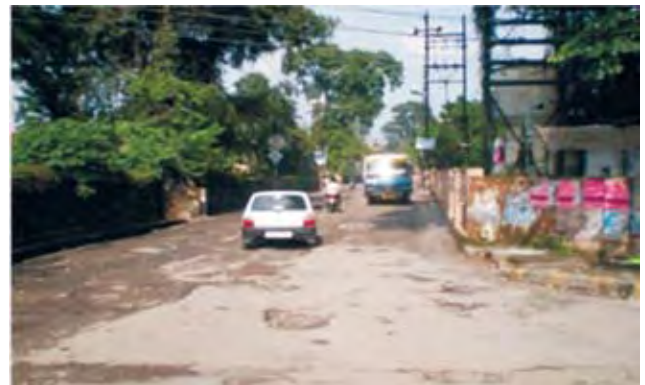
Fig-9 Poor Road Condition
