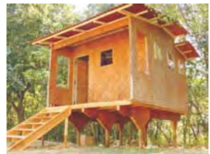
Plate 1 Timber prefabricated Bamboo House
