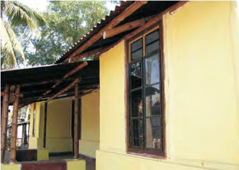
Fig 2. Veranda and Overhang in Demonstration House
