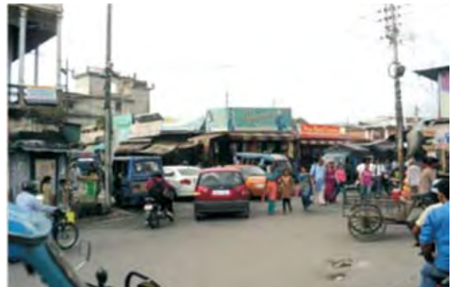
Fig-11 Improper geometrics of junction, Saharanpur chowk
