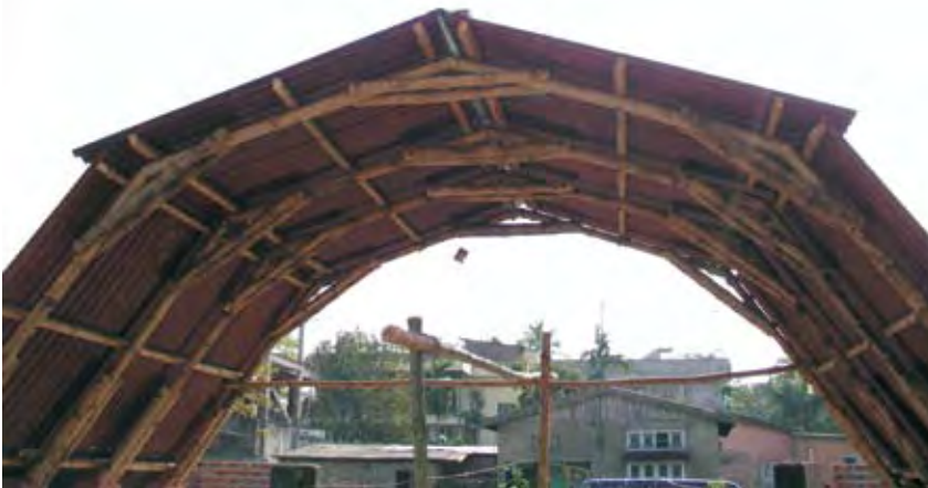
Fig 3. A Bamboo truss being erected
