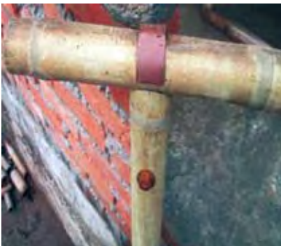
Fig 5. M.S plate joinery for edge beam
