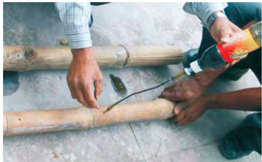
Fig 6. Creosote-Diesel Injection in Bamboo
