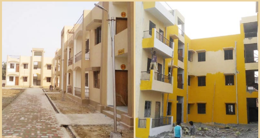
Aurangabad Jagir, Lucknow, Uttar Pradesh [40 DUs (G + 1)] using Stay in Place EPS based double walled panel System (Sismo) – Work has been completed and the project is ready for handing over.
