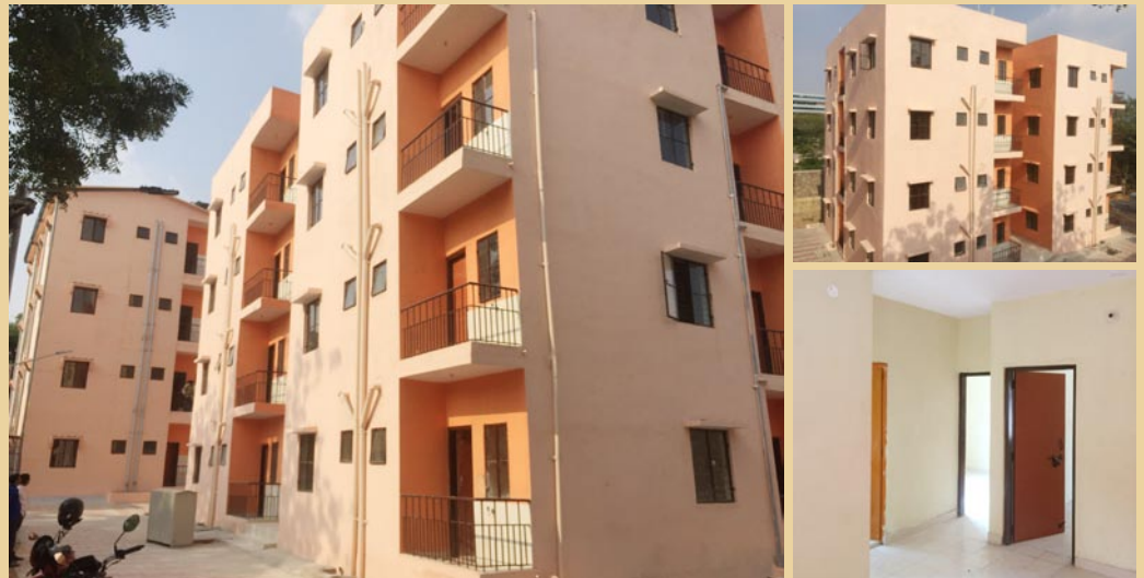
Gachibowli, Hyderabad, Telangana [32 DUs (G + 3)] using Structural Stay in Place Formwork System (Coffor) - 16 DUs and Light Gauge Steel Frame structure (LGSF) - 16 DUs – Work has been completed and the project is ready for handing over.
